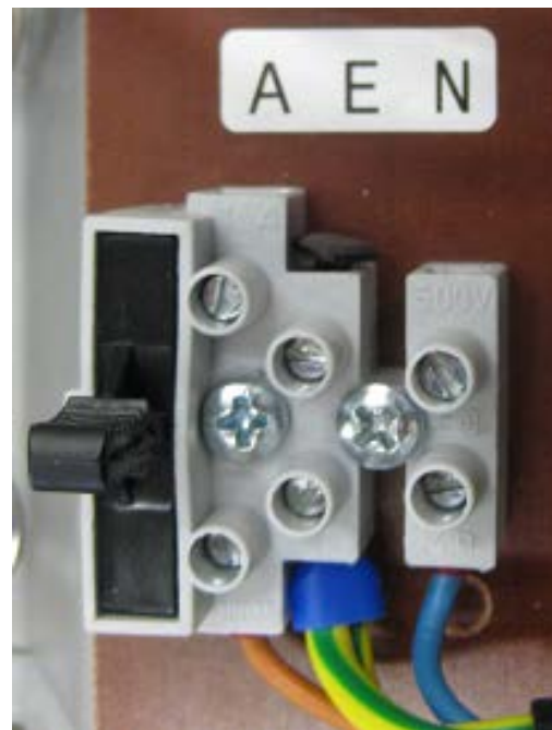
Fused Terminal block (optional)
